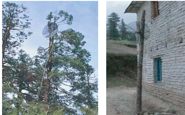
Figure 1 and 2: The antenna for the test to Pokhara from Relay station 1 [left]; and Right: A home built antenna mounted on a wooden pole during the testing period.
